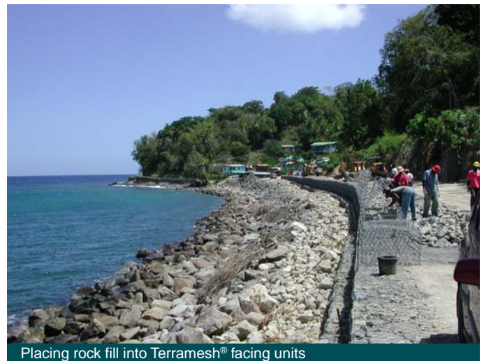
Placing rock fill into Terramesh® facing units
