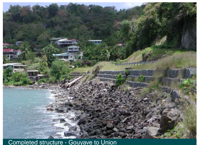
Completed structure - Gouyave to Union
