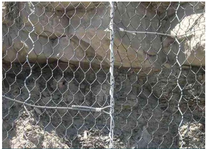
Lacing cable at every mesh opening
