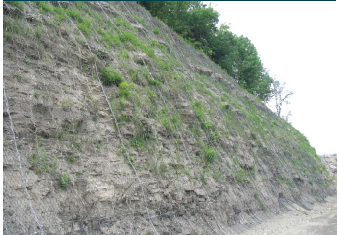
Installed Rock Mesh® B900
