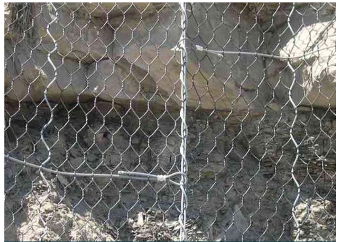
Lacing cable at every mesh opening
