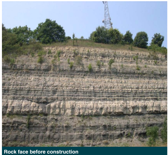
Rock face before construction
