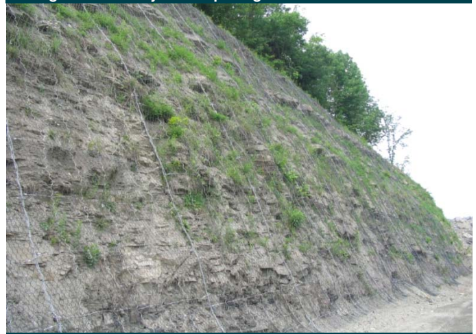
Installed Rock Mesh® B900
