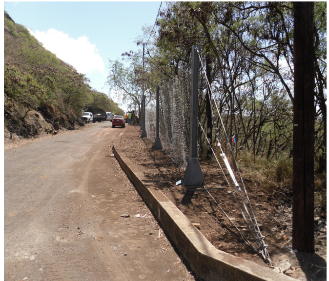
Post Construction: Installed Barrier
