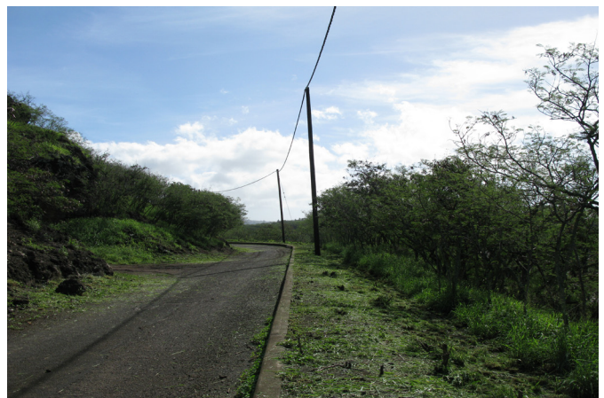
During Construction: Clearing for the barriers
