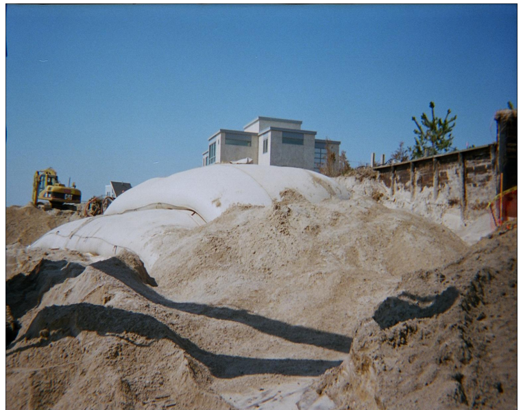
Covering the MacTubes with sand to create the dune
